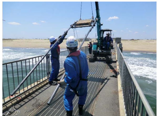
Removal of instrument array.
