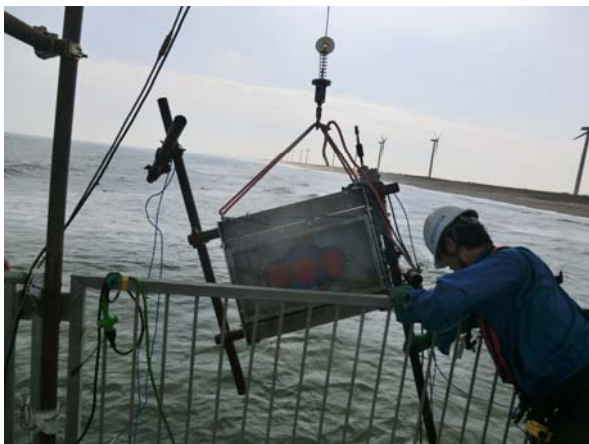
Removal of instrument array
